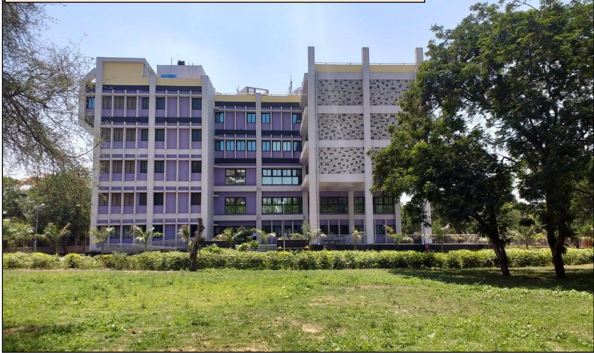
Front view with Green Area of the Office Building
